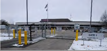
WI-DMA | Whitewater Readiness Center (Armory) Security Gates
